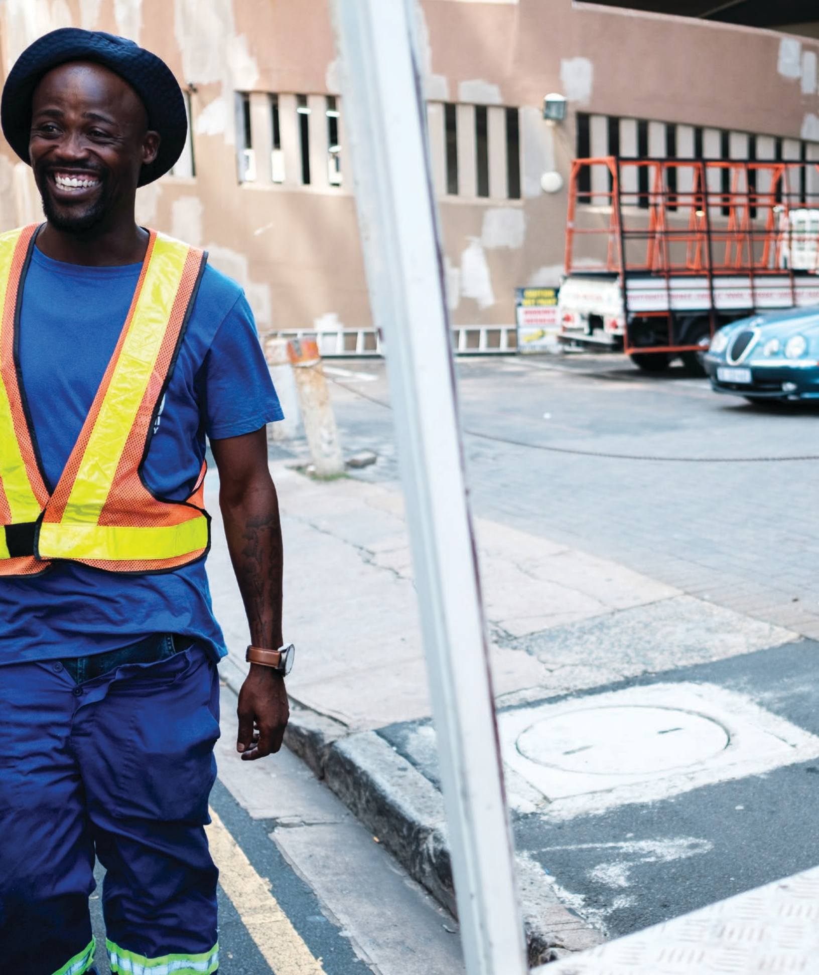
Christopher Magubane (left), 36, and Senzi Dumakude (right), 32, members of an eThekweni Municipality sewage blockage crew at work in Durban. Their team uses flexible rods to clear blockages in pipes leading to the main sewer lines in South Africa, March 2019. © WaterAid / Nyani Quarmyne. Used with permission. Permission required for reuse.
