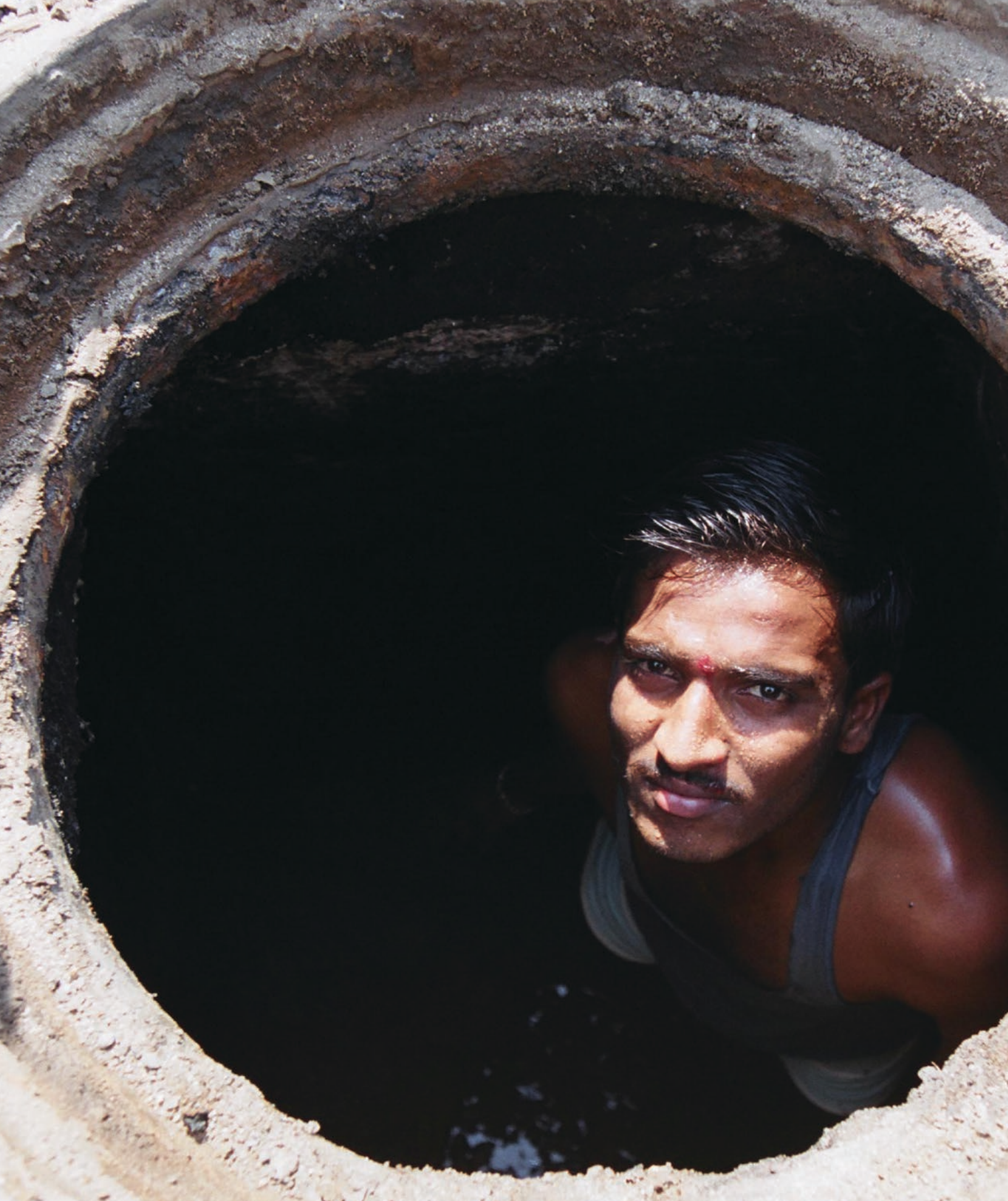
Prakash, sewage worker in Hyderabad, works in the sewer without any protection—no gloves, no suit, no boots. He uses his hands and feet to scrape and clean out the sewage pipes. India, M. Crozet, 2002. © ILO. Used with permission. Permission required for reuse.
